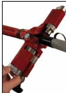
Controlled cut out of the peelable semiconductor sheath
